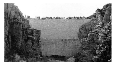
Enterprise Reservoir Dam
