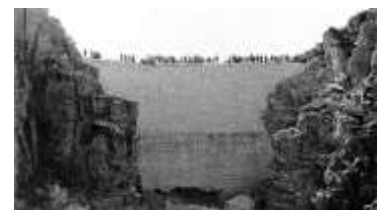
Enterprise Reservoir Dam
